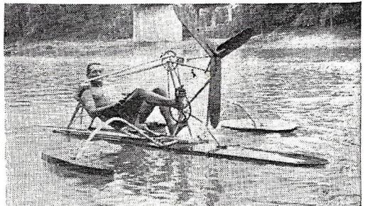
Mounting parts of a bicycle on a surfboard balanced by pontoons, Fred Pilates constructed this novel "aircycle" boat.
