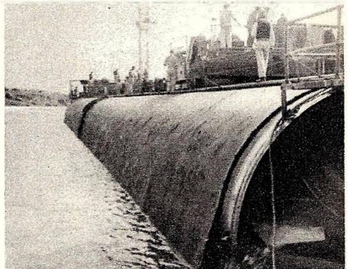
Prepared aboard barges, asphalt sheets are being lowered onto the Mississippi River bottom (above) by U. S. Army engineers in an effort to prevent erosion caused by floods.
