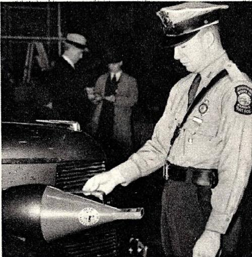
A Kansas highway officer tests the candlepower of an automobile headlight with a portable light-intensity meter.
