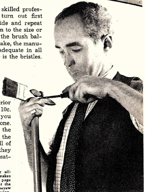
Opposite page—Several types of brushes needed for all-around house painting. Left—A sheet of cellophane makes an excellent moisture-proof holder for a brush. Top of page—The correct way to hold a brush. Right—To paint the inside of a narrow space where the hand can not reach, screw an old brush to the end of a broom handle as an extension.
