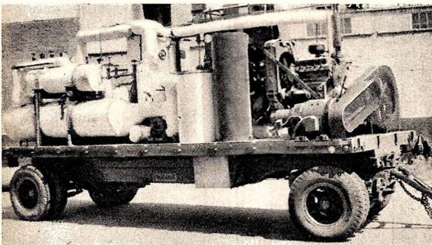
Easily transported from place to place, this complete ice-making unit is capable of making nearly five and one-half tons of ice every 24 hours.
