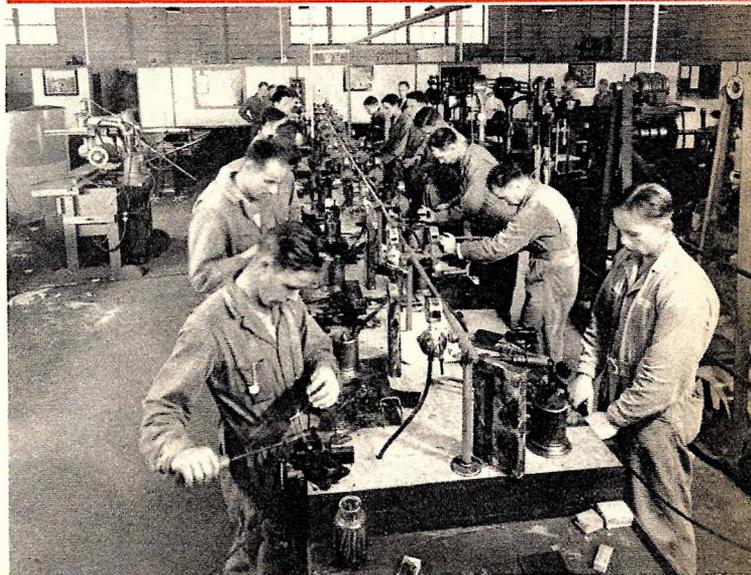
A class in soldering and brazing technique at the Air Corps Technical School, Chanute Field, Ill., is shown in photograph above.
