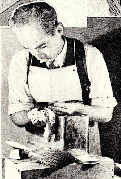
Cleaning a brush immediately after using it will keep it in first class condition for years. Below—A large coil spring will hold the tip of the brush in the paint.
