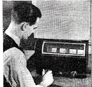
A newly developed parcel post scale (above) can be used to weigh any package up to 70 pounds in weight. In addition, the scale has a calibrated aluminum chart fitted into it in such a manner that as the weight of the package is recorded, the correct figures for postage required to mail the package to various zones is shown.
