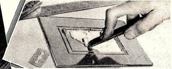
**F**ROM a ten-cent mirror you can make a picture frame that is distinctive and attractive. Remove the backing and the metal or wood surrounding the mirror, and with a pencil mark out the picture opening on the varnish layer that protects the silvering.
