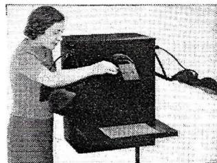
A newly developed portable photocopying machine with a fixed focus makes facsimile copies, similar to photostats, of letters and records and can be operated in ordinary office light.
