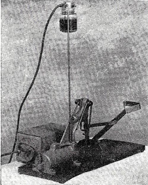
Compressed air for operation of a paint sprayer is created by this foot operated pump. The air is stored in a small tank and released through a regulator valve at a constant pressure.
